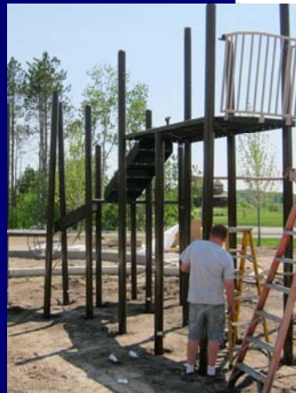
Playground Equipment Installation
