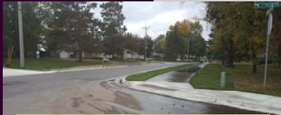
Oneka Lake Boulevard (road reconstruction project)
