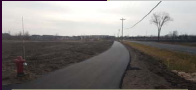
Elmcrest Avenue (residential development)
